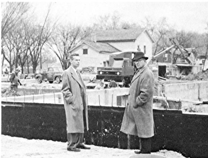
Mr. Bentzin and Mr. Ebert, members of the building committee, keep close watch over the progress of the new high school addition.
