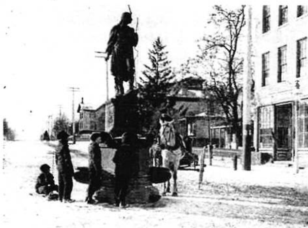
Indian Fountain Horse Trough, cor. Main and Washington Sts.
