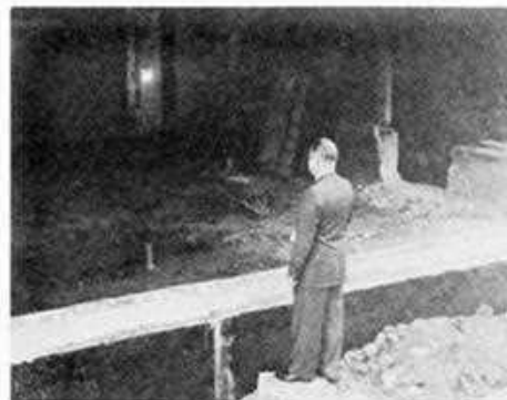
Mr. Stamstad watches progress on the new Band room.
